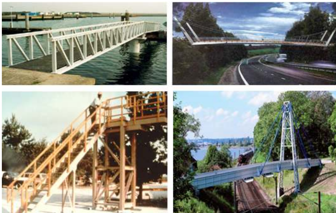
Figure 2. Examples of structure constructed using pultruded GFRP profiles ( www.strongwell.com , 2005)
