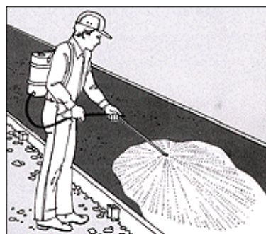
Chemical or liquid membranes reduce evaporation by sealing the concrete.
